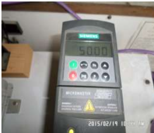
Fig.9 Maximum of frequency on Micro-Master
